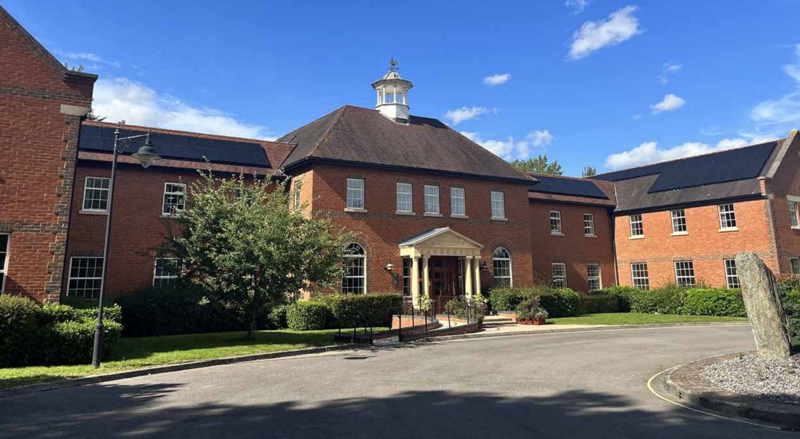
Solar panels installed at Horticulture House in 2023
